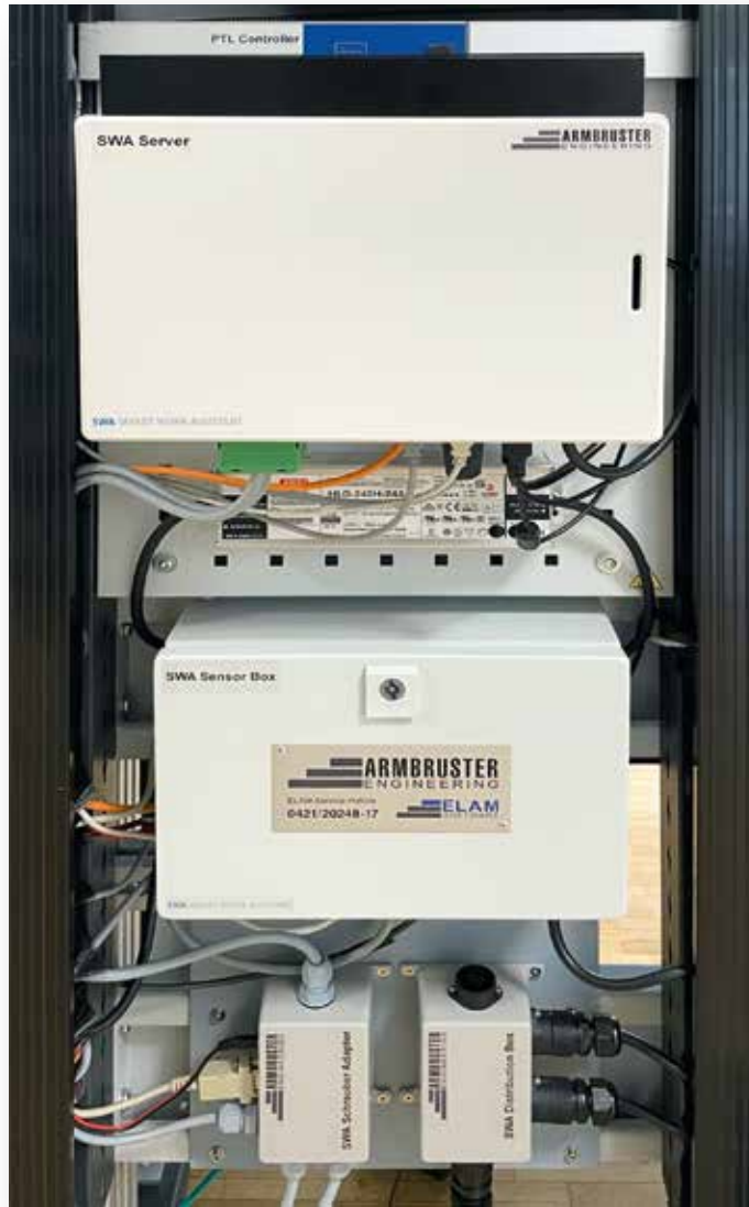
Arrangement of the terminal box with SWA and power unit
